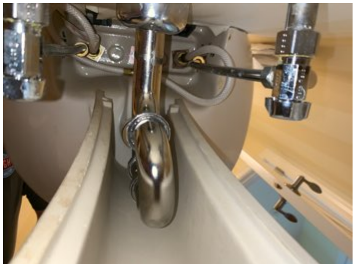
Under half bathroom sink: no leaks observed
