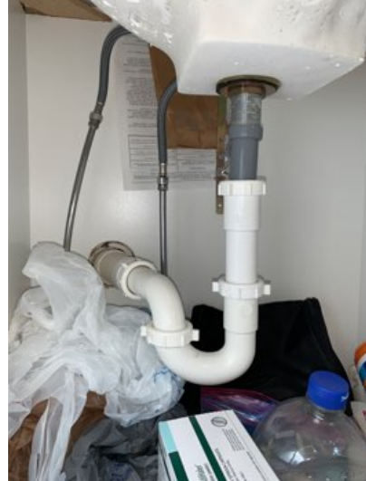
Under bedroom bathroom sink: no leaks observed
