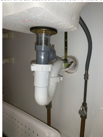
Under Jack and Jill bathroom sink right: no leaks observed
