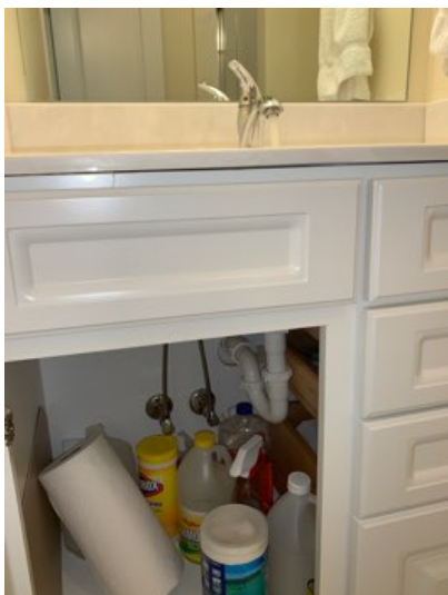
Basement bathroom sink: no leaks observed
