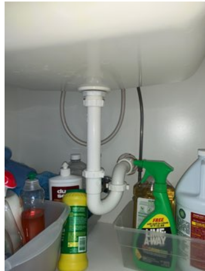
Under laundry sink: no leaks observed
