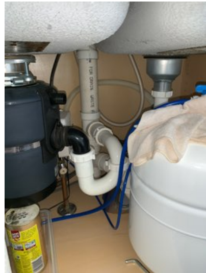
Under kitchen sink: no leaks observed
