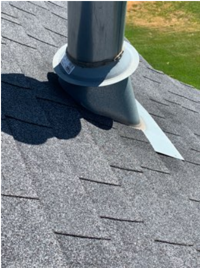
Chimney flashing appears in good condition.
