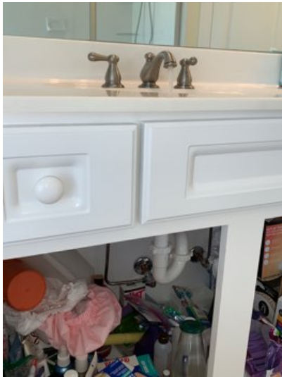
Master bathroom sink left: no leaks observed
