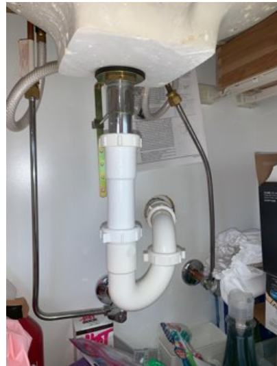
Under master bathroom sink left: no leaks observed
