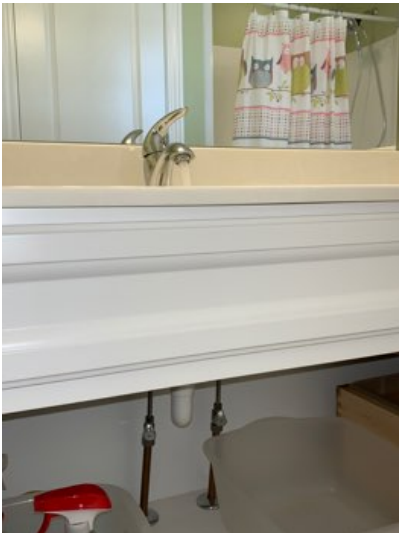
Jack and Jill bathroom sink left: no leaks observed
