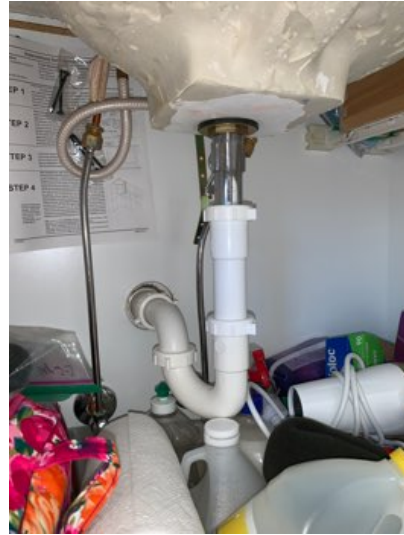
Under master bathroom sink right: no leaks observed
