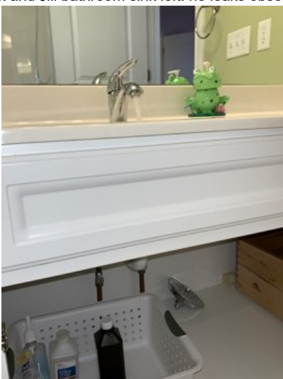
Jack and Jill bathroom sink right: no leaks observed
