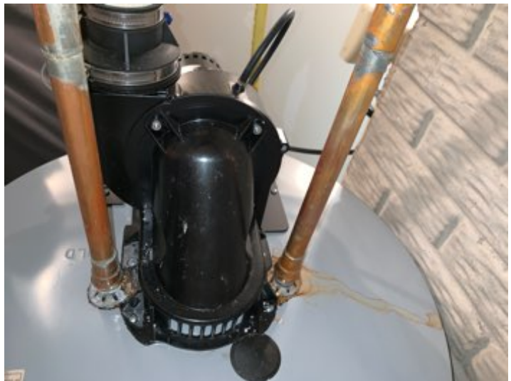
Top of water heater: no leaks, corrosion or damage observed
