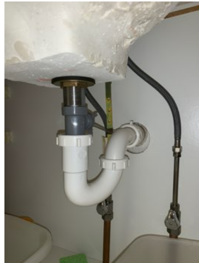
Under Jack and Jill bathroom sink left: no leaks observed
