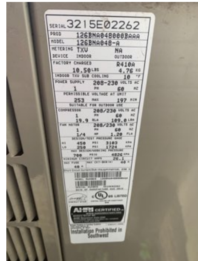
A/C data plate with information and specifications
