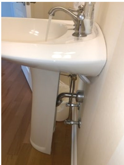
Half bathroom sink: no leaks observed.
