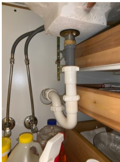
Under basement bathroom sink: no leaks observed
