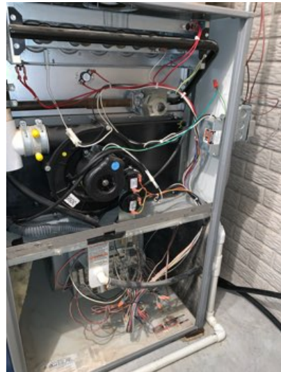
Interior of furnace cabinet: no deficiencies observed.
