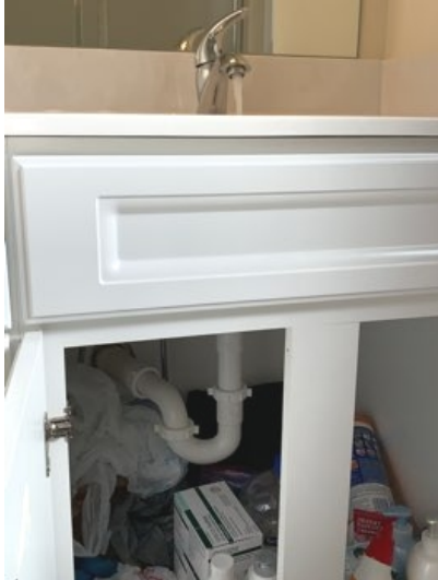
Bedroom bathroom sink: no leaks observed
