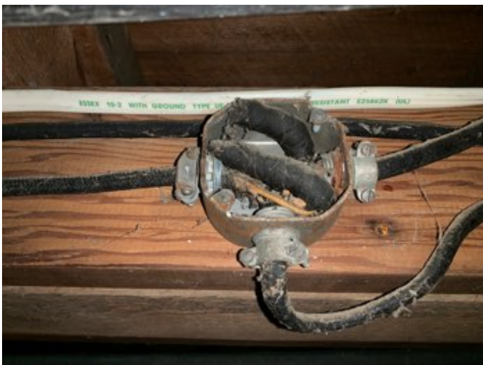
REPAIR - Junction box in the basement were not properly covered. This is improper and less safe. Recommend contacting a certified electrical contractor to assess and repair as needed.
