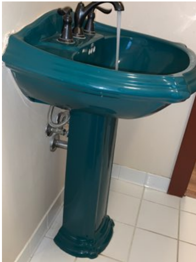
2nd floor bathroom sink: no leaks observed
