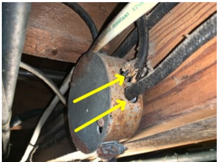
REPAIR - Junction box in the basement were not properly covered. This is improper and less safe. Recommend contacting a certified electrical contractor to assess and repair as needed.
