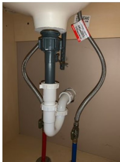
Under 1st floor bathroom sink left: no leaks observed
