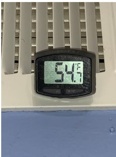
Supply air temperature from Payne A/C unit
