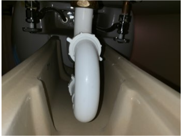
Under 2nd floor half bathroom sink: no leaks observed
