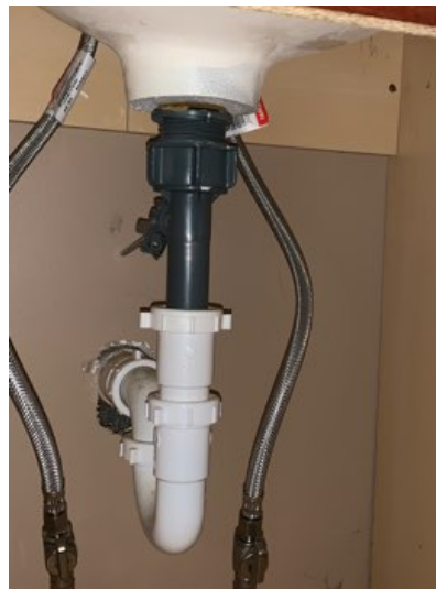
Under 1st floor bathroom sink right: no leaks observed
