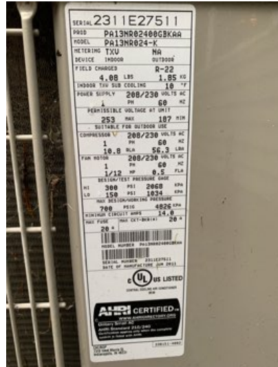
A/C data plate with information and specifications
