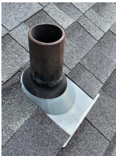
Plumbing stack and flashing appear in good condition.
