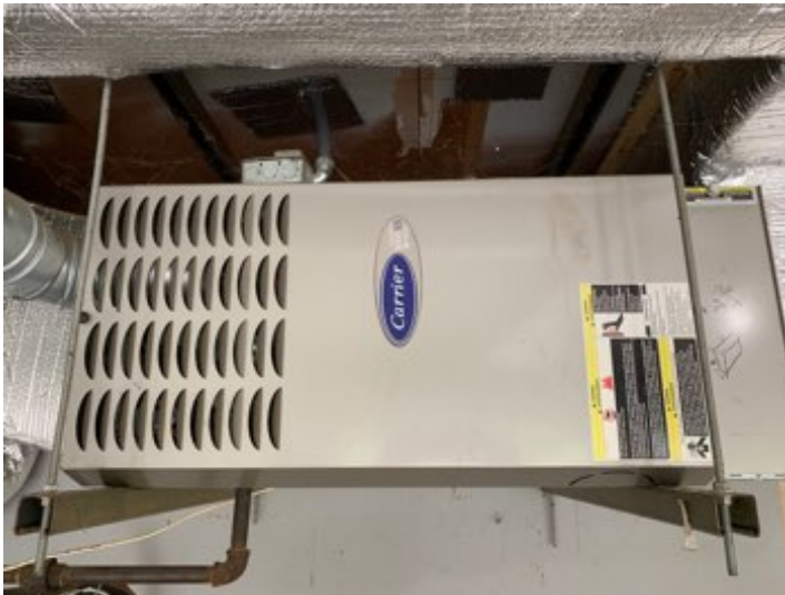
Carrier brand medium efficient furnace
