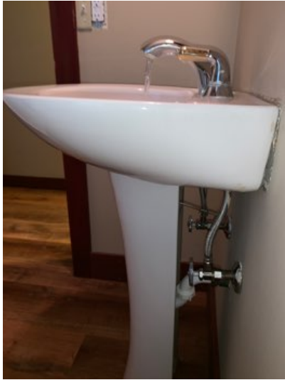
2nd floor half bathroom sink: no leaks observed
