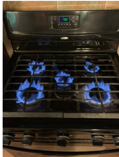
All cooktop burners ignite and appear functional.
