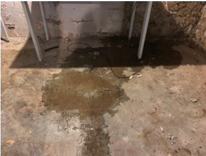
REPAIR- Water/moisture intrusion observed. Water may damage building finishes and structural components as well as aid in the growth of mold. Recommend contacting an appropriate reputable contractor to assess and repair as needed.
