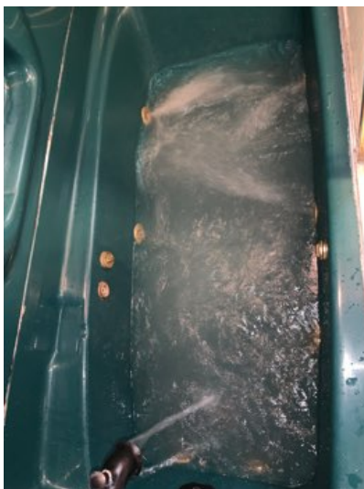
2nd floor bathroom tub
