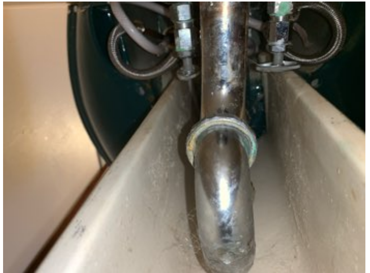
Under 2nd floor bathroom sink: no leaks observed
