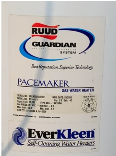
Water heater data plate with information and specifications
