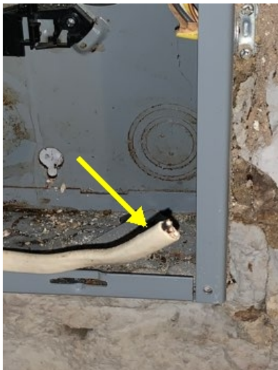
REPAIR- One or more wires in the panel were not terminated properly. This is considered less safe. Recommend contacting a certified electrical contractor to assess and repair as needed.
