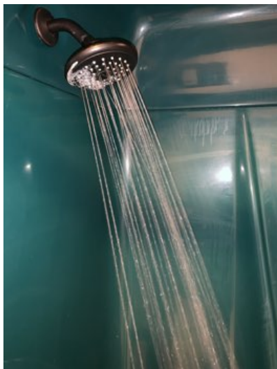
2nd floor bathroom shower
