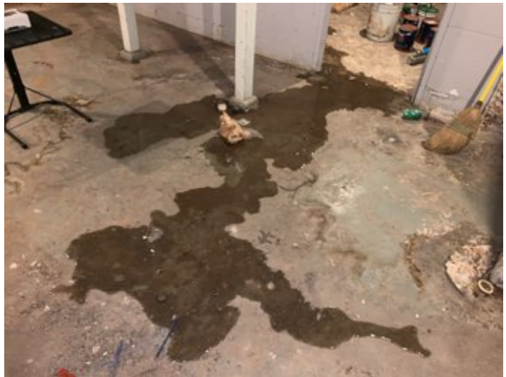
REPAIR- Water/moisture intrusion observed. Water may damage building finishes and structural components as well as aid in the growth of mold. Recommend contacting an appropriate reputable contractor to assess and repair as needed.
