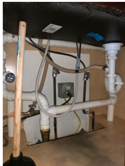
Under kitchen sink: no leaks observed
