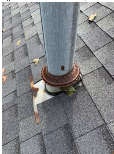
Chimney flashing appears in good condition.
