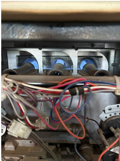
Flames burn bright blue indicating proper fuel combustion.
