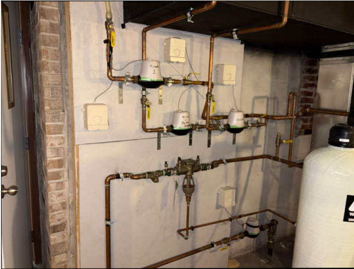
Water meters and shut off valves.
