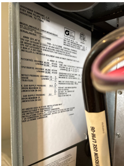
Furnace data plate with information and specifications.
