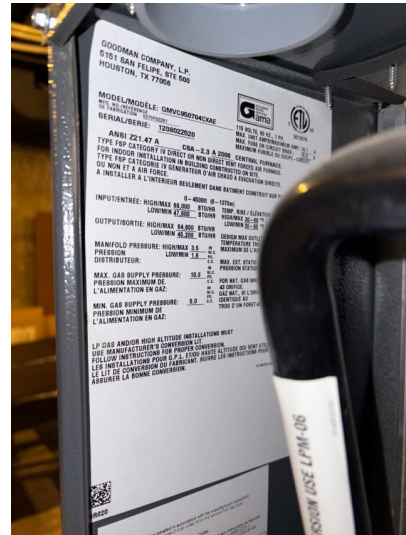
Furnace data plate with information and specifications.
