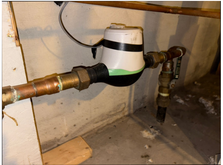
Water supply, meter shut off valve.
